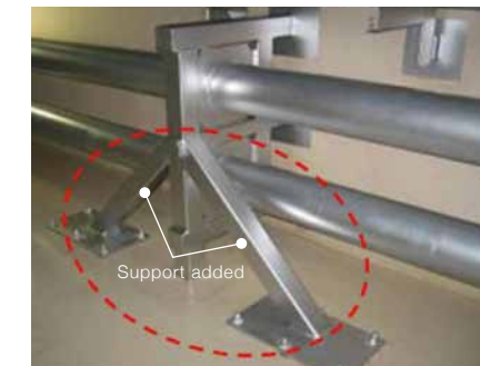
Pipe with support added
