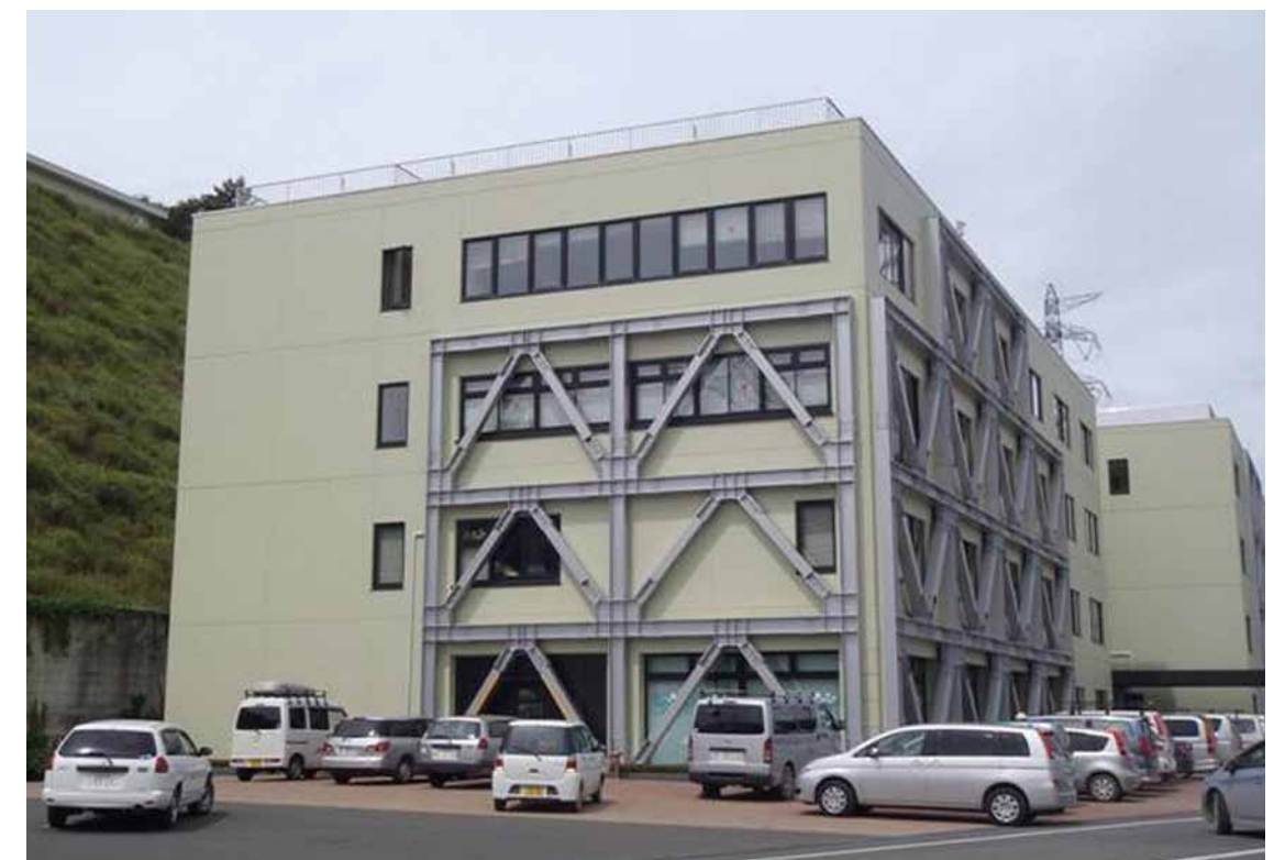
Old administration building that had been reinforced with braces for improved seismic resistance
