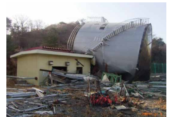
Toppled heavy oil storage tank (Stored amount when toppled: approx. 600kl)
