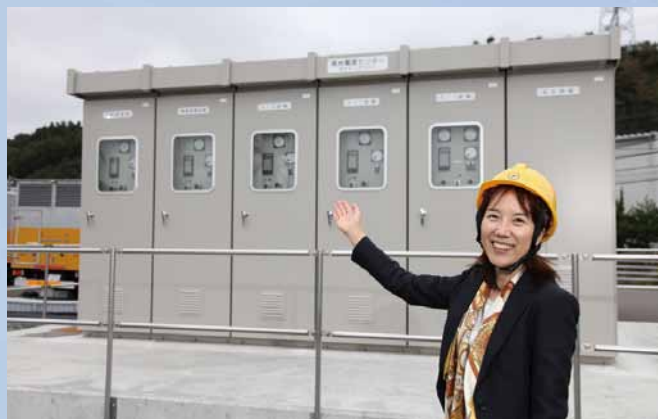
High-voltage power panel in elevated power supply center. Six power supply trucks, able to be connected by cable in an emergency, were also deployed at this elevated site.
